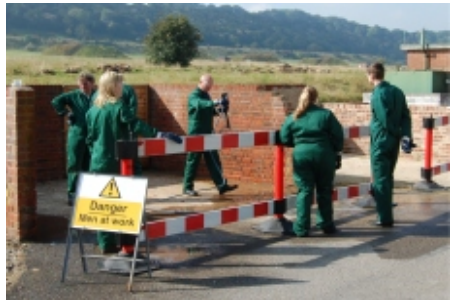
Practising graffiti removal from walls and fences
